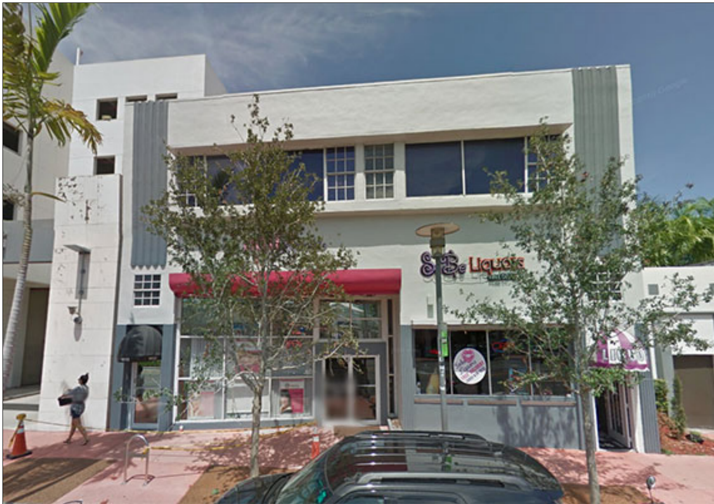
The building at 1609 Alton Road
